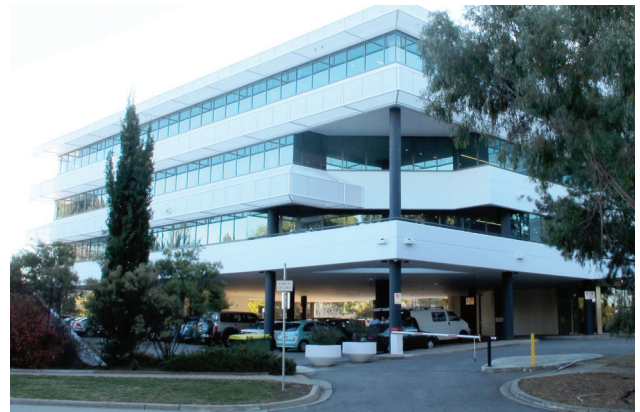
186 Reed Street Greenway ACT Major tenant | Department of Human Services
